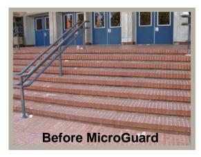
Before - severe staining of brick, grime deeply impregnating mortar, chewing gum hardened on surface and almost impossible to remove.
