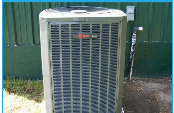
MicroGuard ® coated cabinet after 3 years – clean and shiny with no corrosion.
