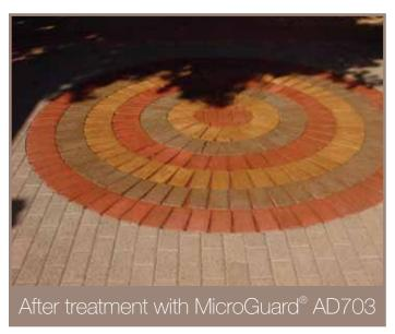
**Situation:** Exterior brick pavers were faded, due to constant sun exposure. The surface was difficult to keep clean. Paver surface was 'dusting' causing a faded appearance.
